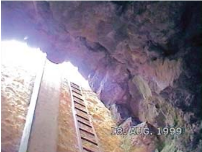
Part of the arch at the rear of the houses (B)
